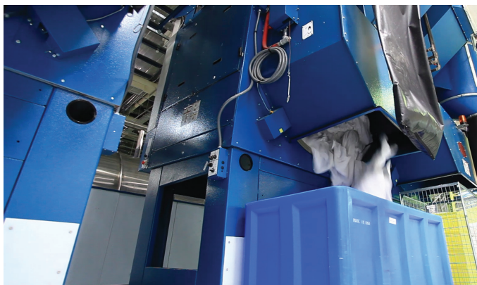
STEAM DRYERS: Milnor supplied its 6458 steam dryers and these are used both for full drying and conditioning
