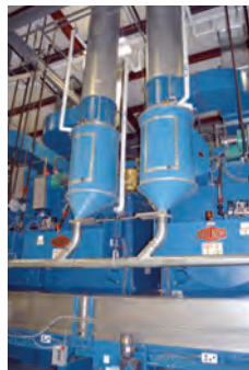
MLF 1010 external lint filter has 36 ft 2 surface area.
