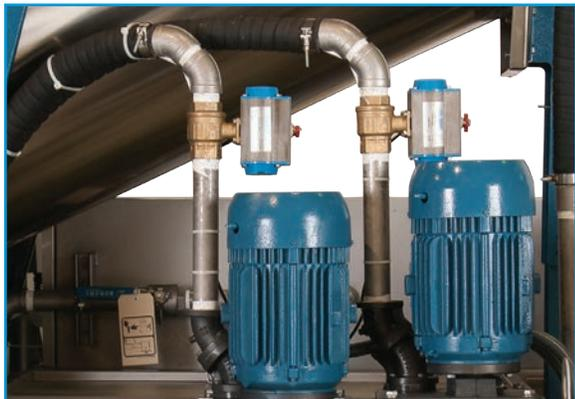
*PulseFlow pumps are specially-engineered for precise process water volume and flow rates which are controlled by electronic flowmeters and inverters.*
