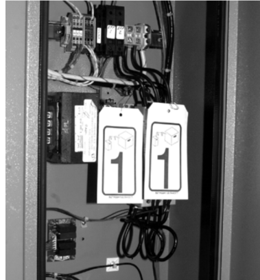
Figure 2. Reconnect Blower Contactor Coil Wires
