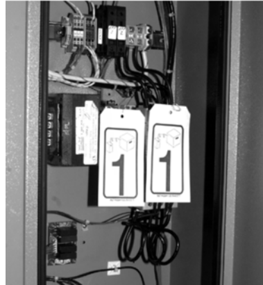
Figure 2. Reconnect Blower Contactor Coil Wires
