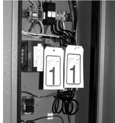
Figure 2: Reconnect Blower Contactor Coil Wires
