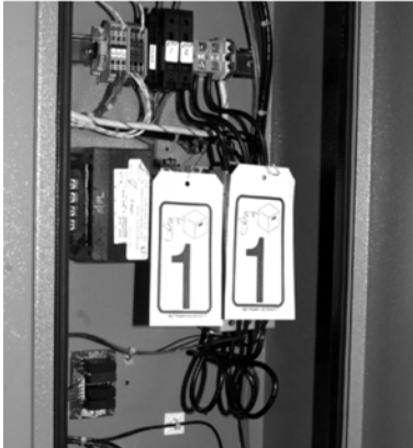
Figure 17. Reconnect Blower Contactor Coil Wires
