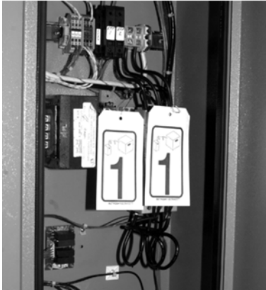
Figure 17. Reconnect Blower Contactor Coil Wires
