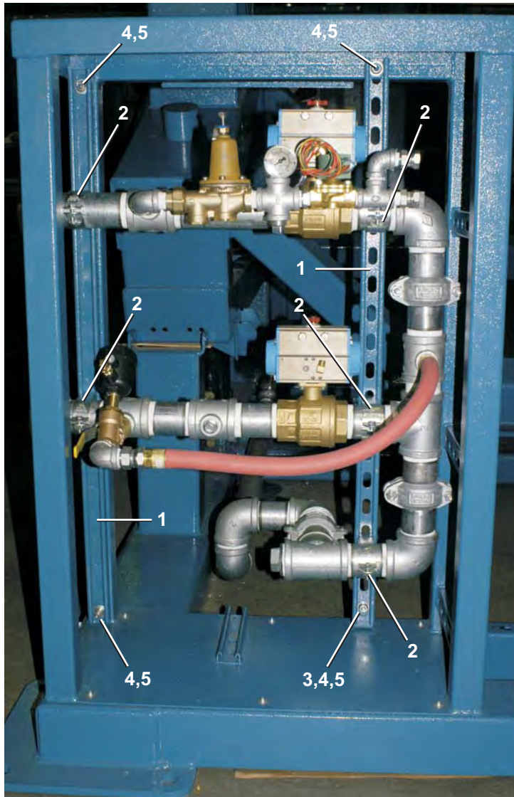
Figure 1: Water valves installed
