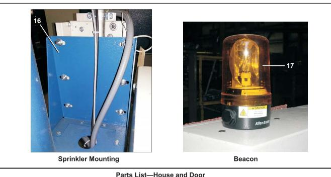
Parts List—House and Door Find the correct assembly first, then find the needed components. The item letters (A, B, C, etc.) assigned to assemblies are referred to in the "Used In" column to identify which components belong to an assembly. The item numbers (1, 2, 3, etc.) assigned to components relate the parts list to the illustration.
