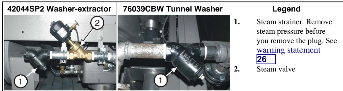
Figure 12: Steam Inlet Strainer. These are examples. Your machine can look different.
