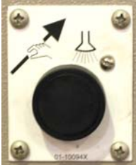
Figure 7: Manual Supply Flush button
