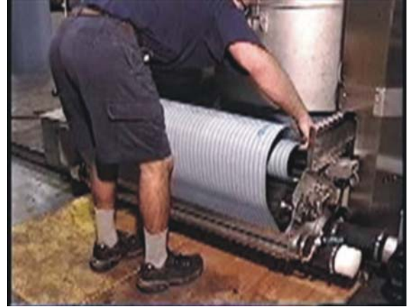
Figure 30: Pulling Belt Through Press from Unload End
