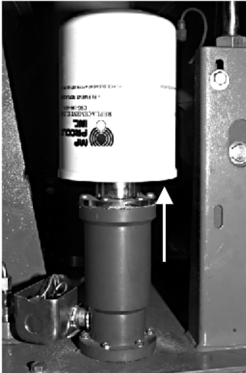
Figure 8: Breather/Moisture Filter
