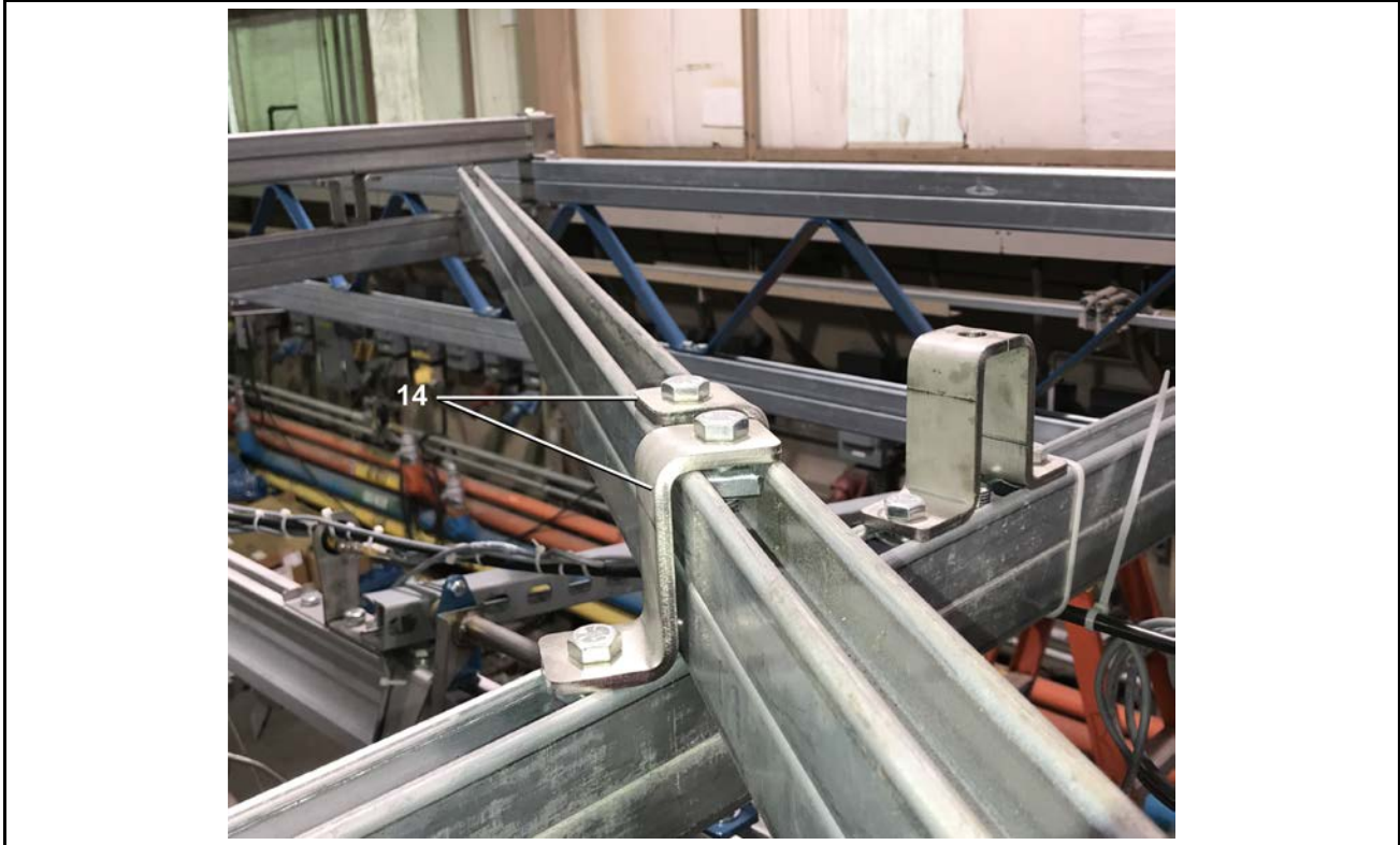
Figure 9. Additional Unistrut Beam Connectors
