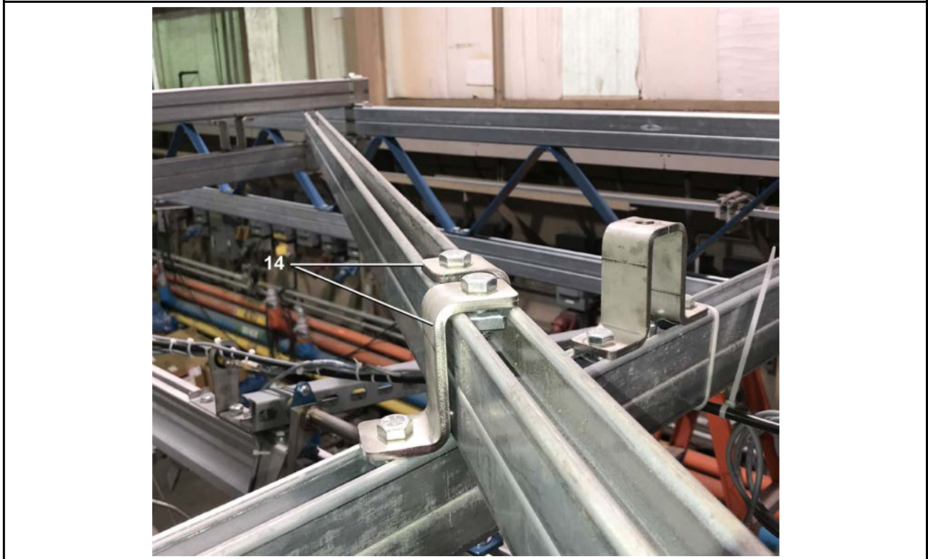
Figure 9. Additional Unistrut Beam Connectors
