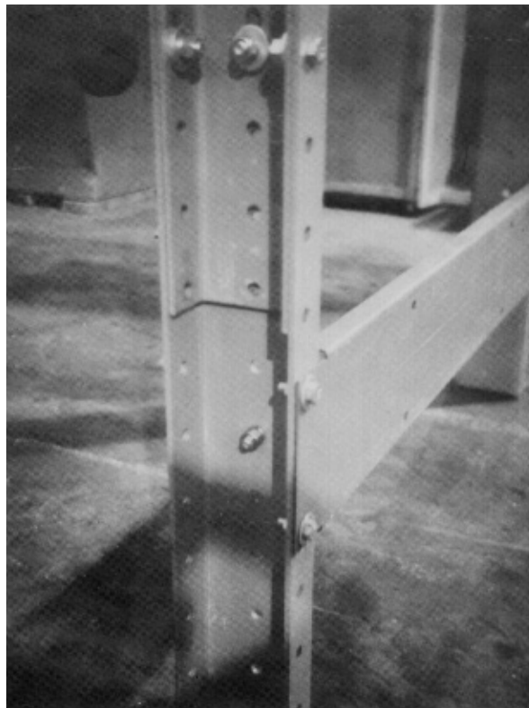
FIGURE 5: Crossmembers, one of two shown.
