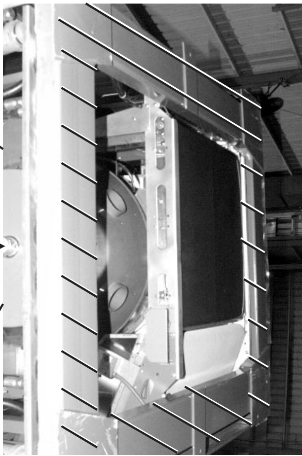
FIGURE 2 (MSINA406AE) Lifting and Jacking Points
