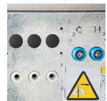
Safe chemical injection
