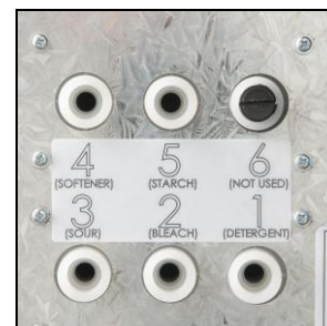
Safe chemical injection
