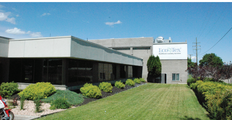
GREEN ASPECT: The future is green inside and out at Ecotex - Kelowna. The laundry was designed to service 80 healthcare facilities scattered geographically in the interior region of British Columbia
