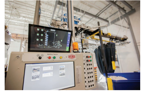
KEEPING UP: The Milnor system has been operating for a year with nearly 100% uptime
