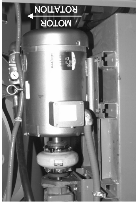
FIGURE 11 (MSSMA423AE) Hydraulic Pump Rotation
