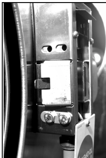
Figure 2: Adjustment bolts removed, showing slotted adjustment
