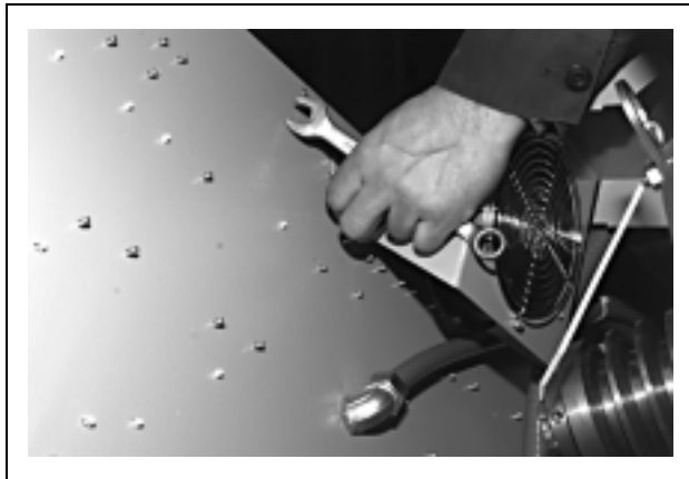
FIGURE 7 (MSSM0285AE) Removing Fan For Hoist Clearance
