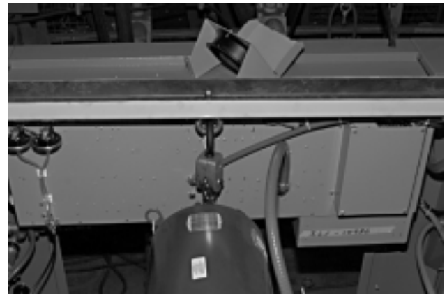
FIGURE 8 (MSSM0285AE) Bearing Support Fixture in Place
